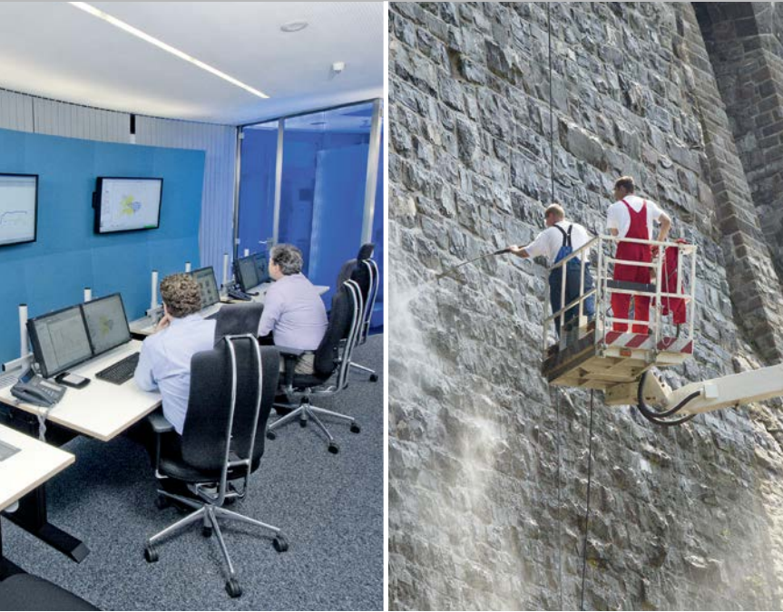
View of the Reservoir Control Centre (left), cleaning of the masonry dam (right).
