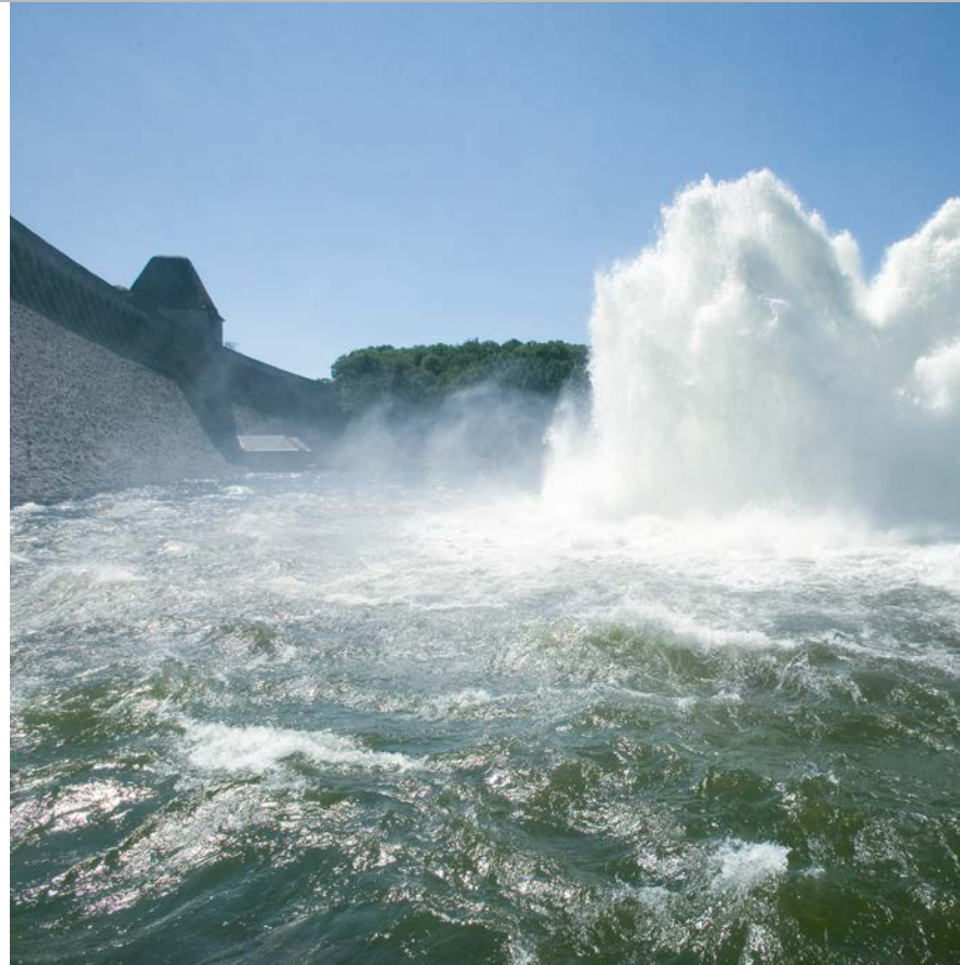
The bottom outlets are being tested for proper functioning.
