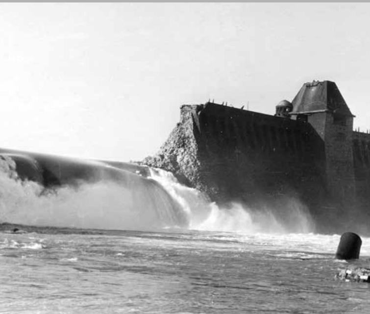
Water streamed from the reservoir through a 77 metres wide gap.
